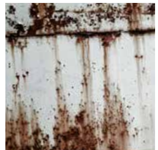
Preventing rust and corrosion
